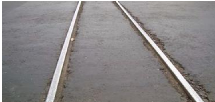
Gambar 3. 29. Rusak Perpotongan Rel ( Railroad Crossing )
