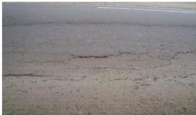
Gambar 3. 9 Cekungan ( Bumb and Sags )
