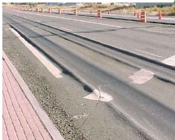
Gambar 3.30 Alur ( Rutting )
