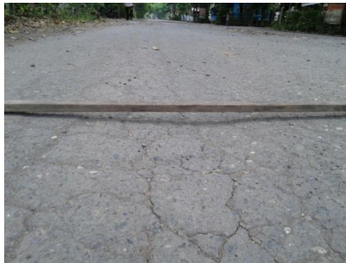
Gambar 3.8 Cekungan ( Bump and Sags )
