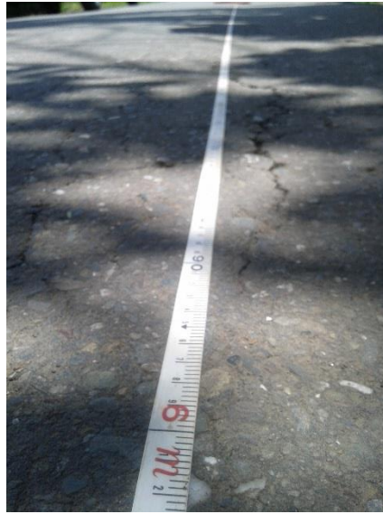
Gambar 3.24 Pengausan Agregat ( Polised Agregat )
