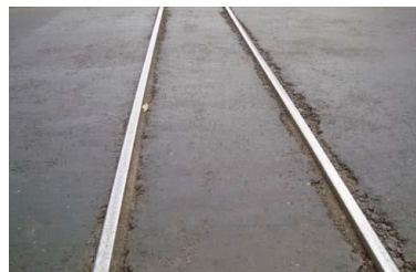
Gambar 3.28 Rusak Perpotongan Rel ( Railroad Crossing ) Sumber : Bina Marga No.03/MN/B/1983
