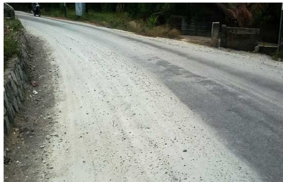
Gambar 3.38 Pelepasan Butir ( Weathering/Raveling ). Sumber : Bina Marga No.03/MN/B/1983
