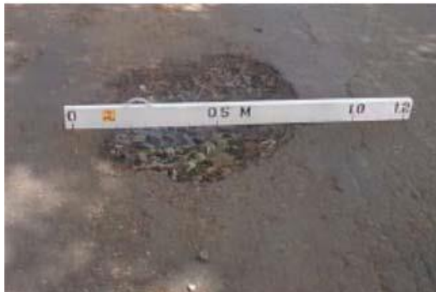
Gambar 3.26 Lubang ( Pothole )
