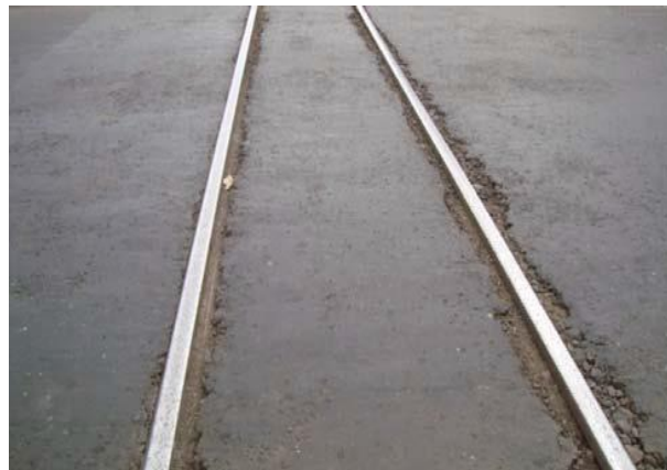
Gambar 3.28 Rusak Perpotongan Rel ( Railroad Crossing )
