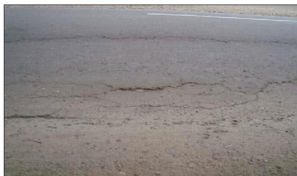
Gambar 3.8 Cekungan ( Bump and Sags )
