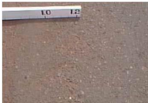
Gambar 3.24 Pengausan Agregat ( Polised Agregat )
