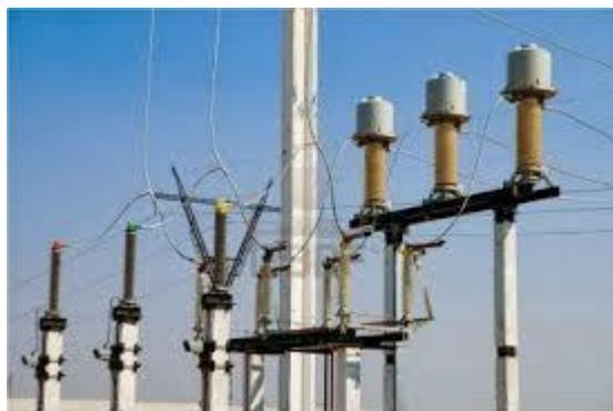
Gambar 2.13 Pemisah (PMS)/ *Disconnecting Switch* (DS)
