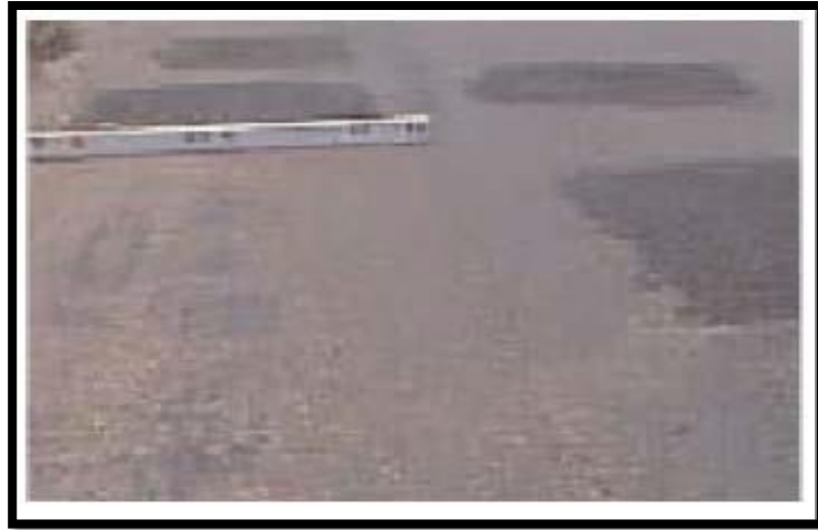
Gambar 3.23 Tambalan ( Patching end Utiliti Cut Patching )
