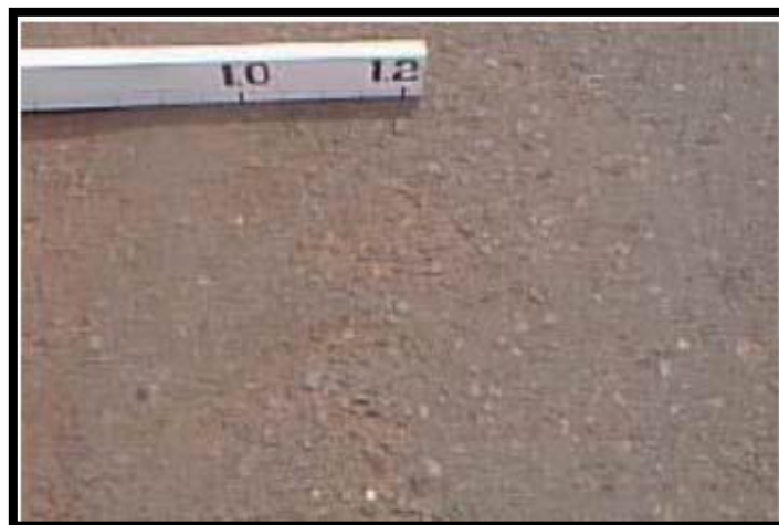
Gambar 3.25 Pengausan Agregat ( Polised Agregat )
