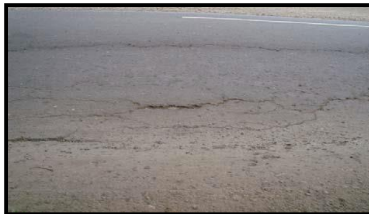
Gambar 3.9 Cekungan ( Bump and Sags )
