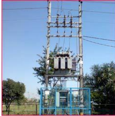
Gambar 2.5 Transformator Distribusi
