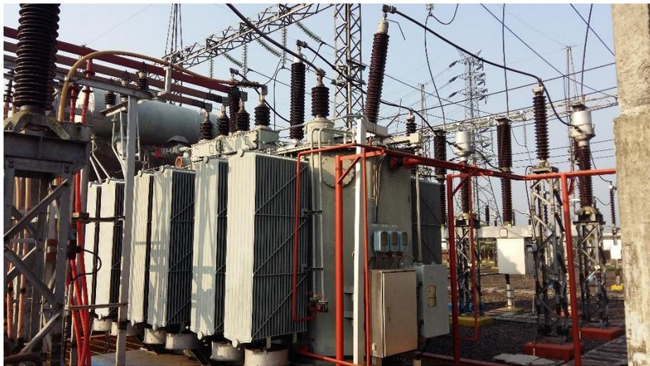
Gambar 2.2 Transformator Daya
