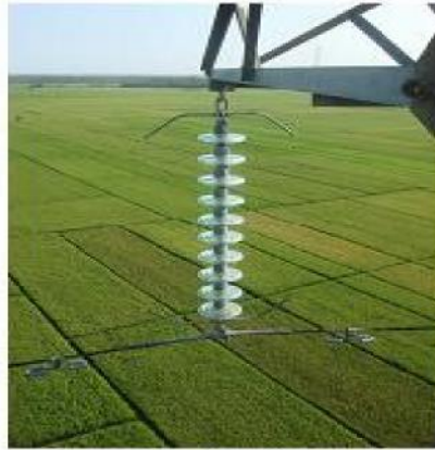
Gambar 2.7. Isolator piring
