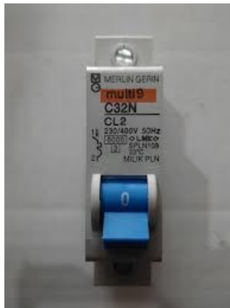
Gambar 2.16 MCB ( Miniature Circuit Breaker )
