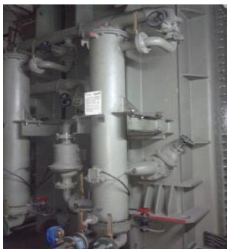
Gambar 2.13. Pendingin Transformator
