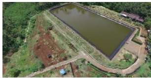
Figure 2: Aerial looks over Embung Abimanyu
