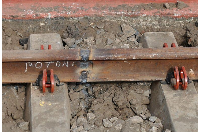
Gambar 3.3 Continuous Welded Rails
